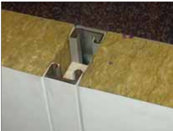
Figure 16: Insulated core panels – internal panel
